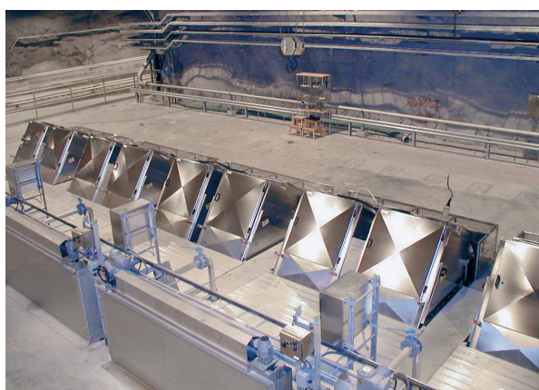
Meva Rotoscreen in a WWTP
