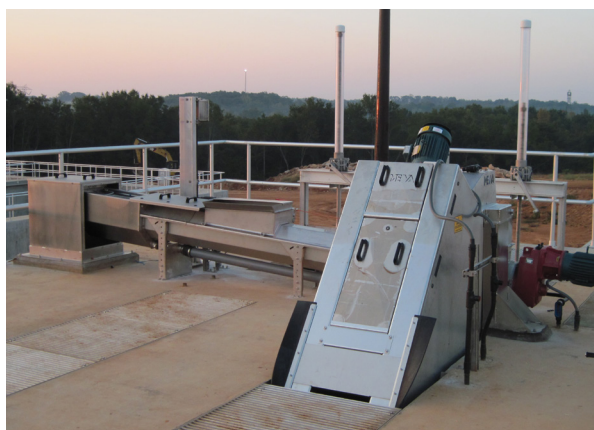
Meva Rotoscreen - fully capsulated
