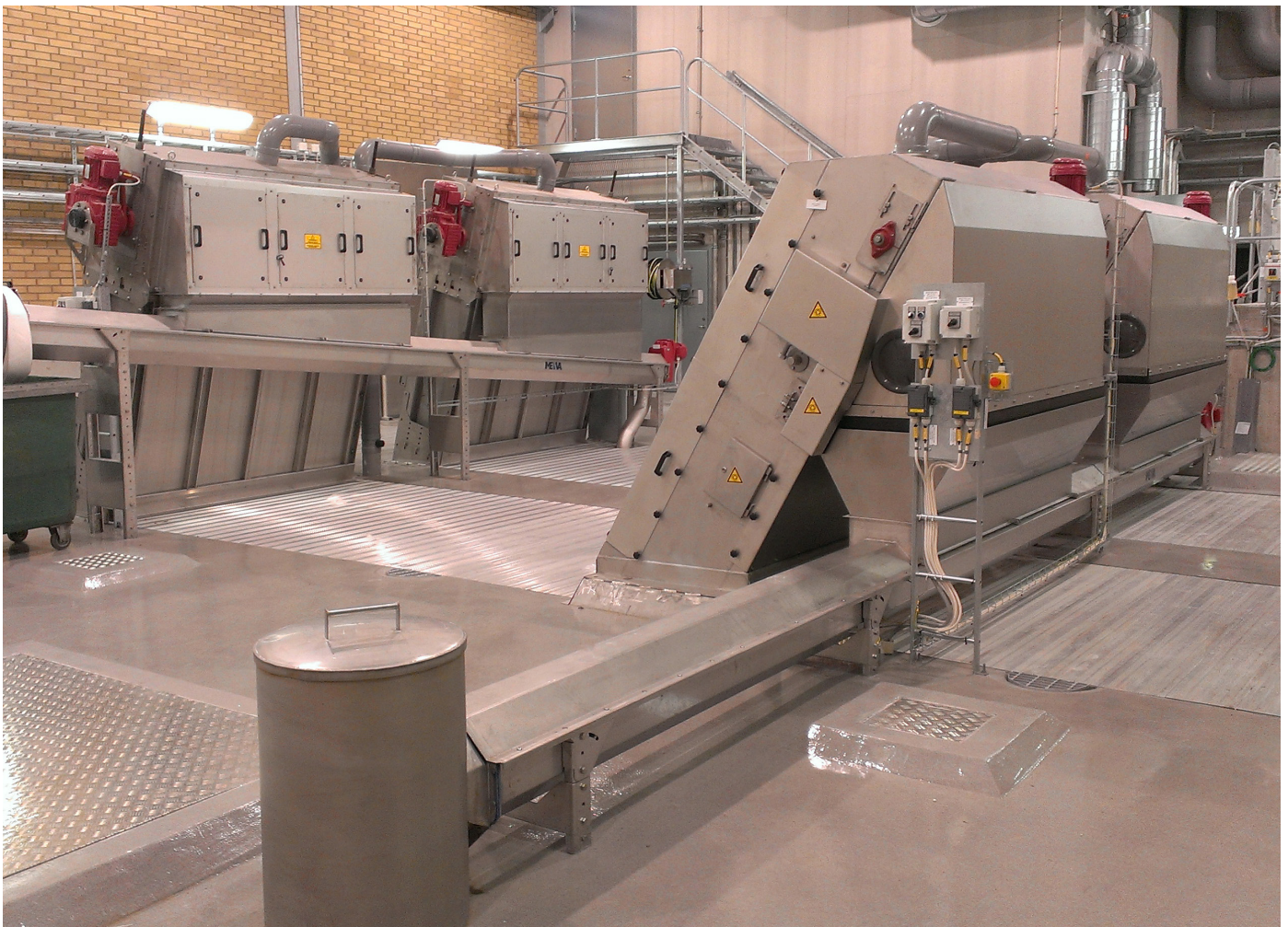
Meva MPS with Meva MRS coarse screens and XC spiral conveyors
